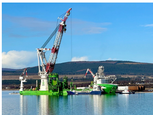
Orion working on Moray West
